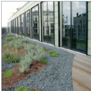
Roof terrace and facade
