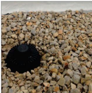
Roof, terrace and facade
