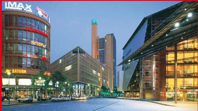
ACO surface drainage at Potsdamer Platz, Berlin
