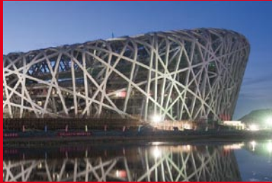
ACO drainage systems for the Olympic stadium in Beijing
